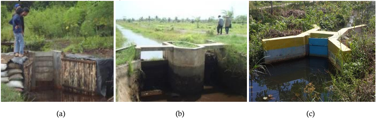
Gambar 5. Model tabat dari kayu (a), beton (b), dan flap gate (c) Figure 5. Tabat model from wood (a), cement (b), and flap gate (c)
